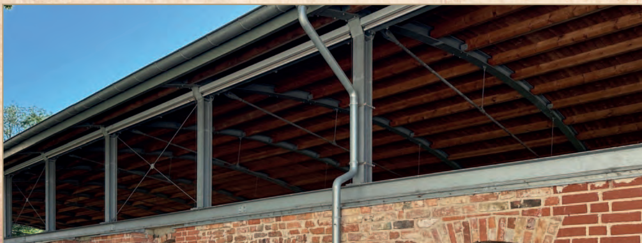
Weather protection roller blinds – Altfriedland Monastery Ruins
